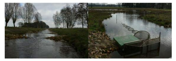
Figure 19. The shallow V notch pass Kaweise Loop (left, 12-03) and the upstream inlet of the fish siphon pass with fish trap and coupling piece (right, 12-03)
